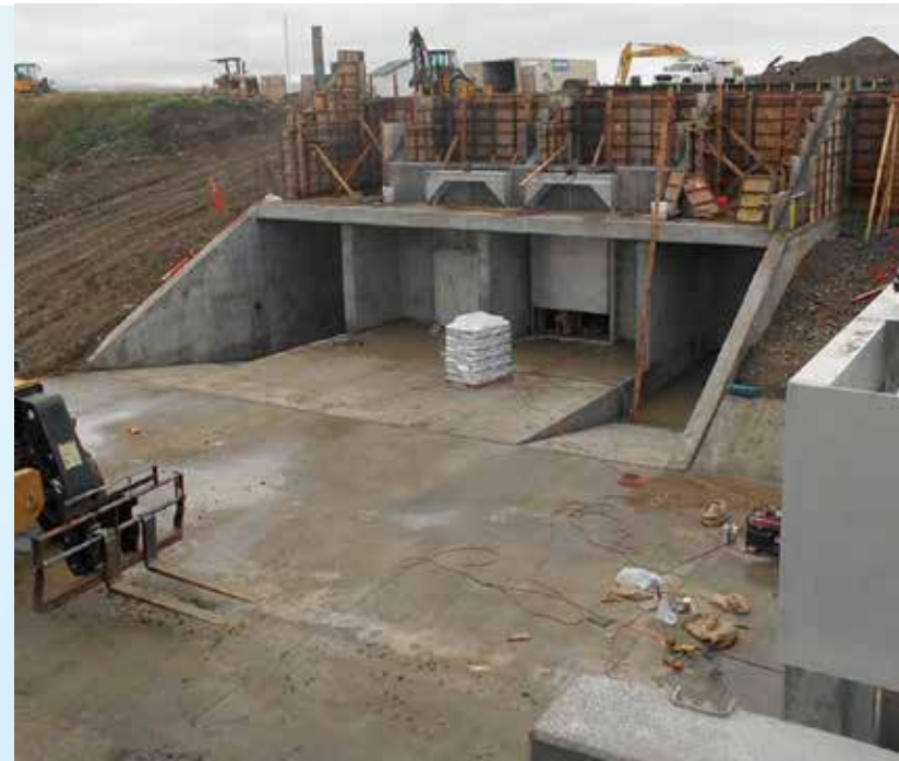
Los Banos Creek Weir and Diversion Construction
