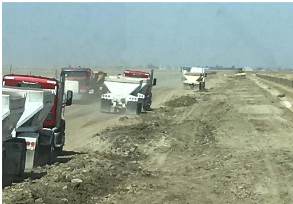
Placement of sediment in reuse area
