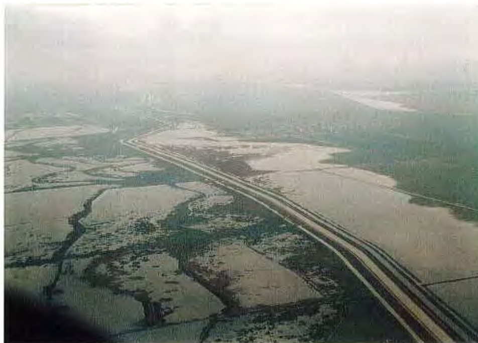
2/10/98 LOOKING EASTERLY ALONG MAIN CANAL AND MAIN DRAIN FROM CAMP 13
