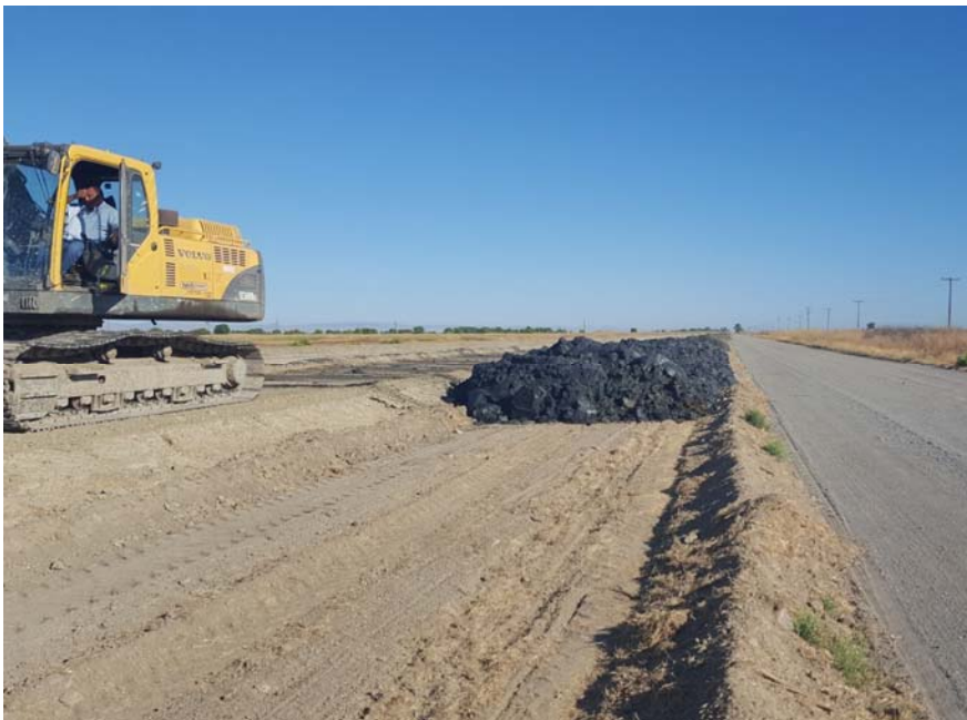
Placement of sediment prior to loading in trucks
